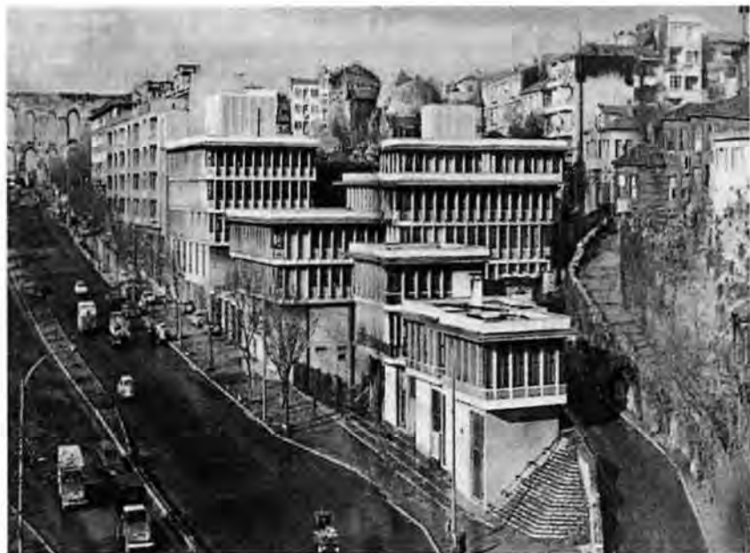
Figure 8.8. Social Security Agency Complex, Zeyrek (Sedad Eldem, 1962-1964), Istanbul. (Aga Khan Trust for Culture)
